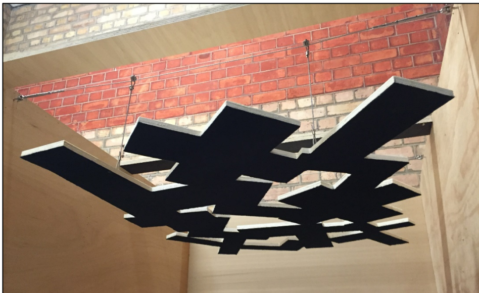
Figure 4: The prototype of the acoustic 'cloud' panels. Photo: Contractor, Janus and Patel (2016).
